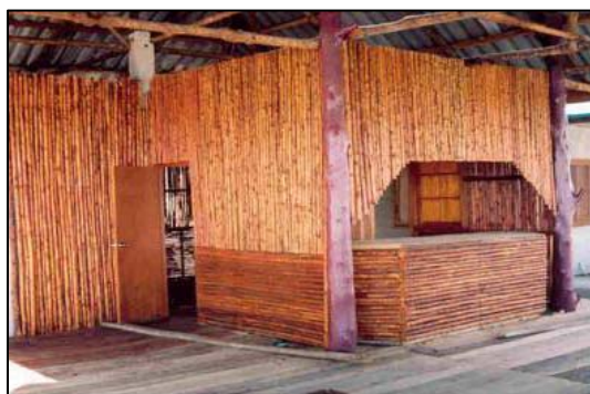
Thinned wood of Rhizophora apiculata is used to build houses in Can Gio, HCMC (Source: MERD)
